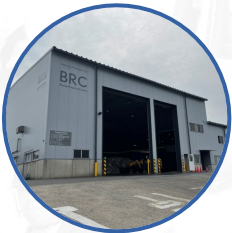
BRC Plant (Beverage Container Recycling)
